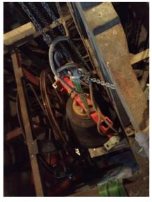
the Bellhanger e m p l o y e d b y Nicholson Engineering he, Chris and Robin, were able to 'thread' the 300kg bell up through them, thereby saving a lot of additional work. By 7:30 in the evening the replacement bell was installed, the old bell secured firmly in place, the re-bushed clapper to the treble fitted, and new ropes
